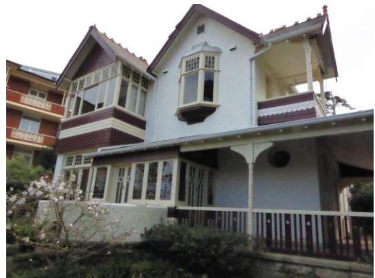
Figure 40: Front (south) elevation showing later (c.1911) infill to front verandah and balcony at first floor level
