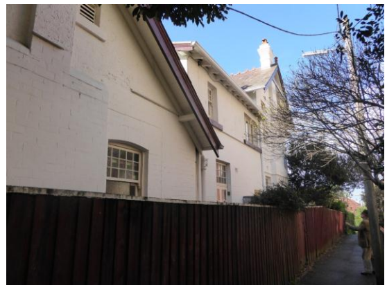
Figure 42: Side (west) elevation showing roof forms of the separate wings.
