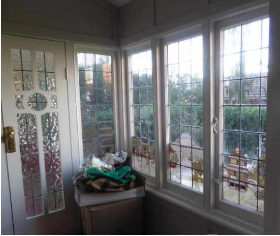
Figure 67: Early 20 th century addition of enclosed verandah at ground level with stained glass windows in 'Asian' theme
