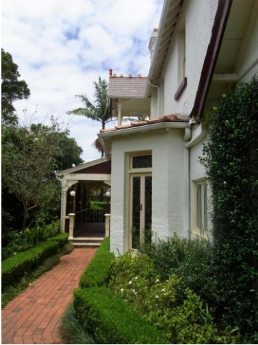
Figure 43: Side (east) elevation showing projecting bay window with front verandah in background
