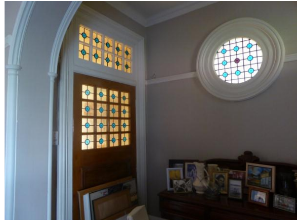
Figure 64: Leadlight oriel window, highlight and panels to door from entry vestibule into Sitting Room
