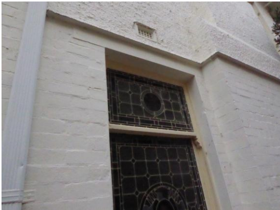
Figure 51: External view of leadlight window to dining room showing evidence that it is a later opening containing a relocated window.
