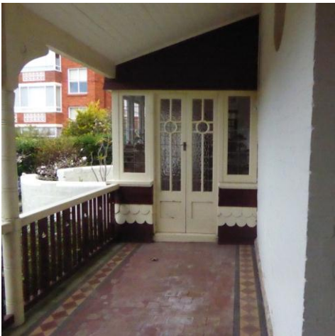
Figure 45: Front verandah showing entry to later enclosed verandah section
