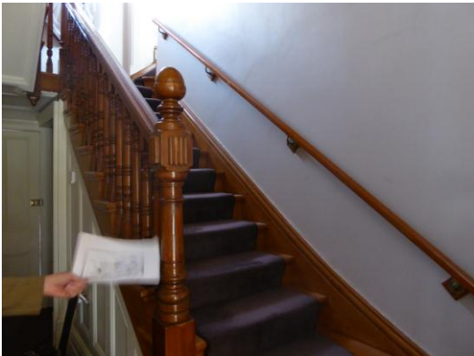
Figure 75: Original timber stair
