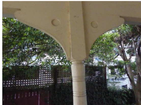
Figure 48: Detail of turned timber posts and brackets
