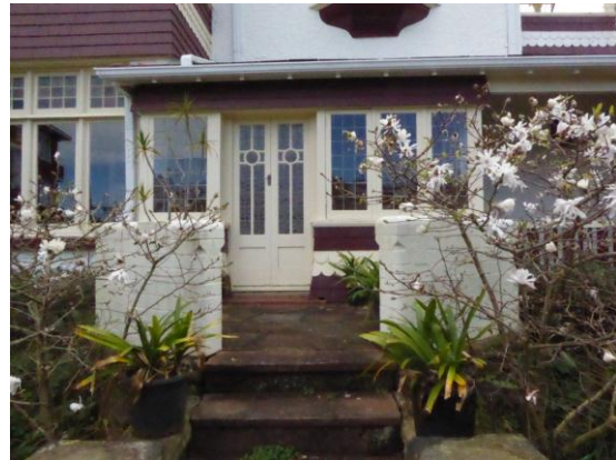
Figure 46: Entry steps leading to later addition enclosed verandah
