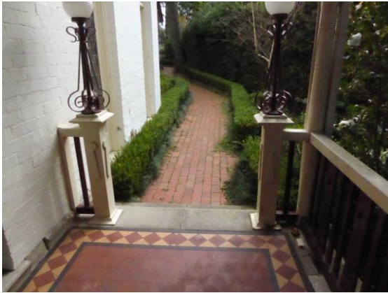
Figure 49: Relocated timber posts and relocated light fittings to north end of verandah
