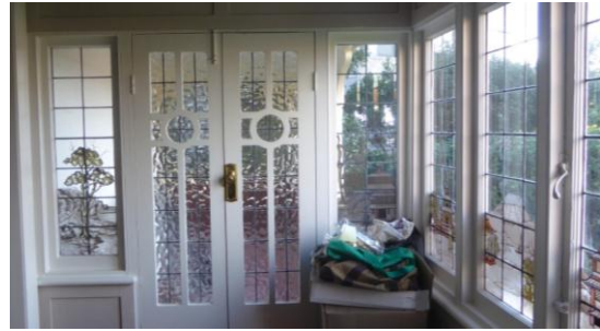
Figure 68: Early 20 th century addition of enclosed verandah at ground level with stained glass windows in 'Asian' theme
