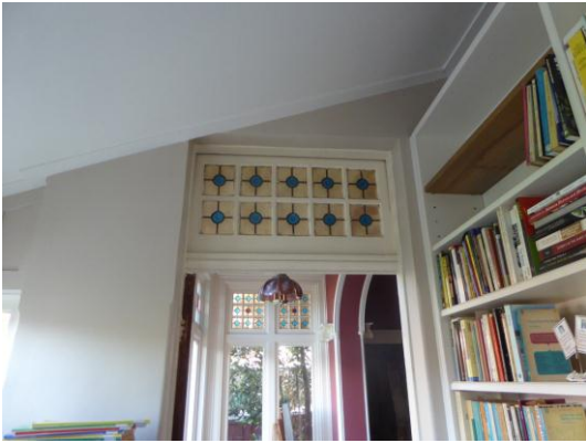
Figure 73: Leadlight glazing to highlight above door to original enclosed verandah
