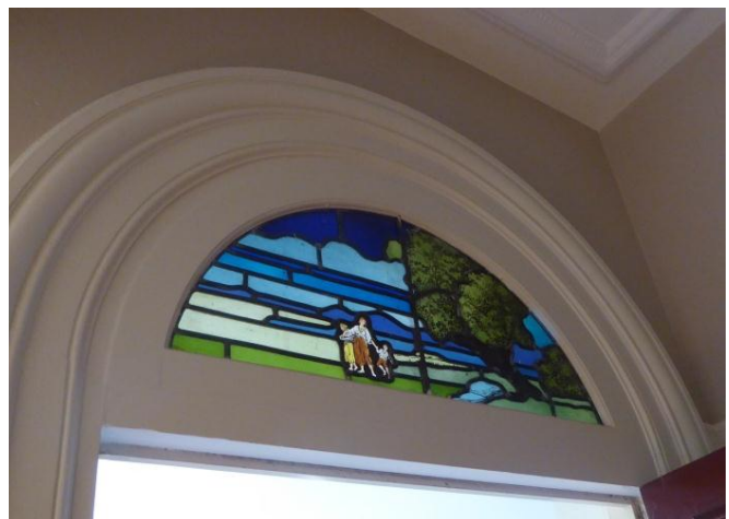
Figure 54: Fan light to front door with original lead light
