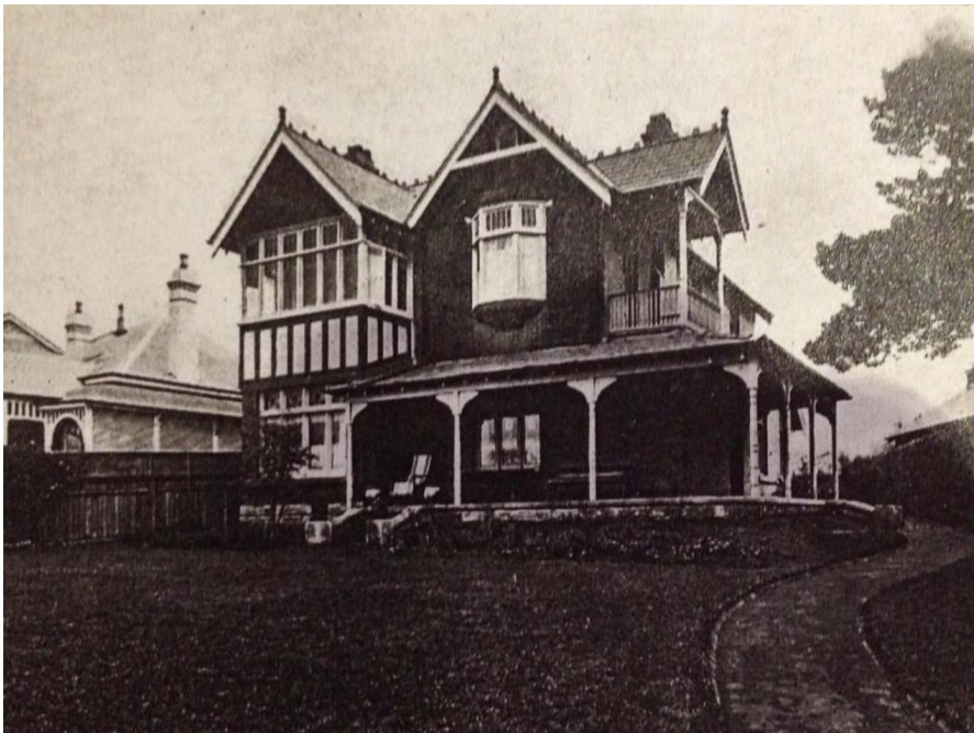
Figure 24: Extract from BA 546/228 showing rear (north) elevation and side (east) elevation of the rear wing with addition of bay window and alterations to original/early windows. (Source: North Sydney Council archives)
