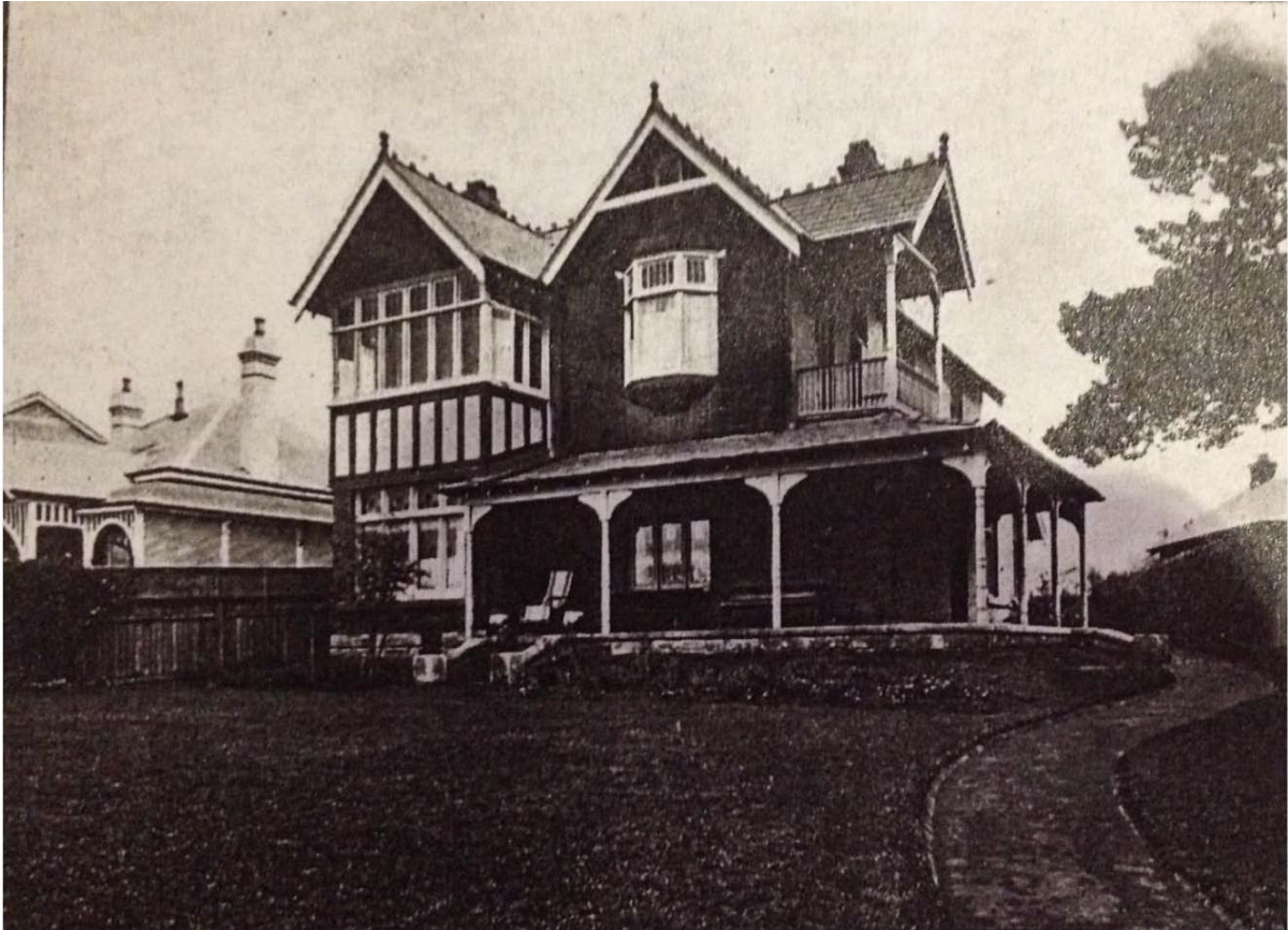
Figure 13: Photograph of Lansdowne, 3 Raymond Road in 1919 from the Property and Premises Journal (1 st September 1919). The caption for the image read: “‘Lansdowne’, Neutral Bay, a Fine Residence, possessing Distinction in Architecture and Site.” Note that at this time, the enclosed verandah on the front elevation had not been constructed.
