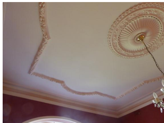
Figure 72: Original ceiling, cornice and ceiling rose to Dining room
